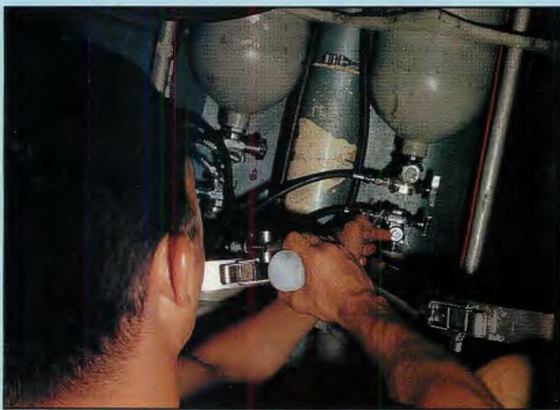
UDT-21 Petty Officer Putnam uses soapy water to check for leaks in his team's SCUBA regulators prior to 1973 dive. Solution bubbles over an air leak. A malfunctioning breathing regulator could injure or kill a frogman.
