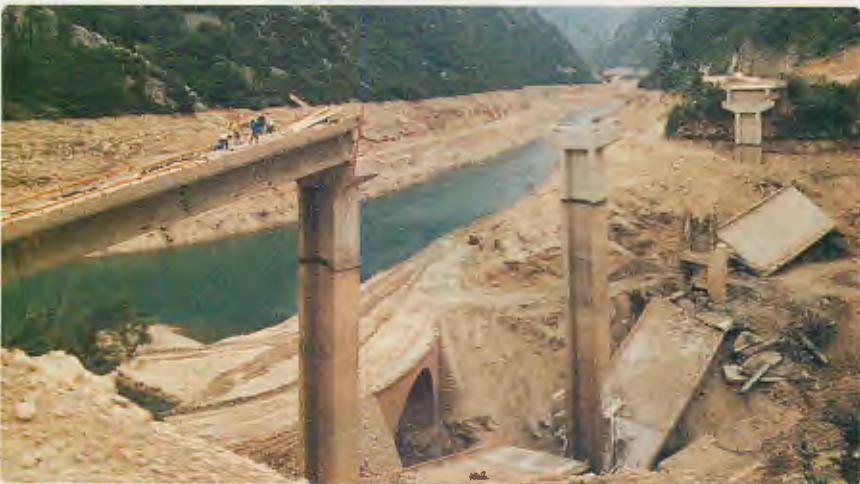
Major destruction was encountered along most of the route into Sarajevo with bridges and other infrastructure just now being rebuilt.
