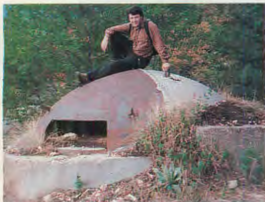
Author rests atop small bunker — one of roughly 176,000 built — guarding a road into the capital city of Tiranë. Some bunkers, such as this one, incorporated steel sheathing.
