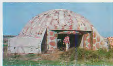
Larger bunkers, such as this one on hill south of Tiranë which overlooked road to the sea, could accommodate crew-served weapons. Weathering-giraffe paint job was intended to be camouflage. Albanians now use many of these larger bunkers as living quarters and businesses.
