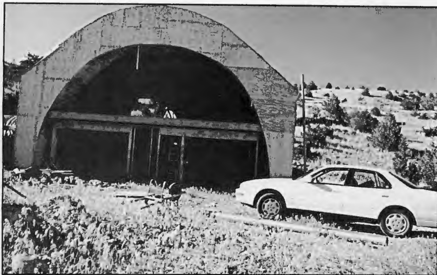
Car gives perspective on concrete- and steel-reinforced Quonset hut-shaped structure, reported by TV news as designed for storage of APCs purchased by Prophet's church. As shown, building is too small for such use and is actually a residence under construction, with part of home built into hillside. Photo: James L. Pate
