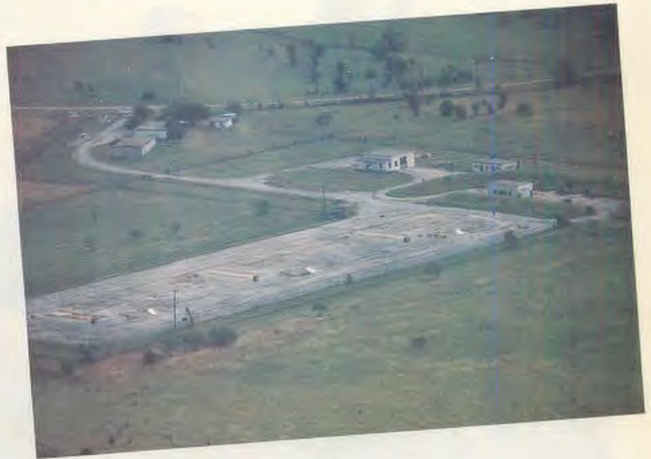
Looking to the northeast by air, entrances can be seen to the 15,000 square feet of underground facilities. At right are the ordnance area and building, utilities building and test lab, and at left is the bomb shelter and residence.
