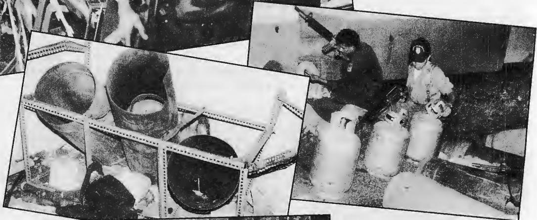
**ABOVE:** Salvo soldiers inspect captured *Tepescuintle* components. At right are LPG tanks modified to be launcher tubes; center are smaller LPG tanks that comprise explosive projectiles; at left are improvised plywood obturating discs, propellant charges, and bags of cement used to stabilize tubes for firing.
