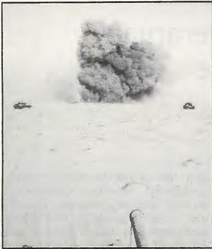
1st Bn. combat engineers shooting line charge into first minefield inside Kuwait. The charge is a chain of 1,100 pounds of C4, rocket-assisted. Photo: 1st Lt. Brian Hornberg
