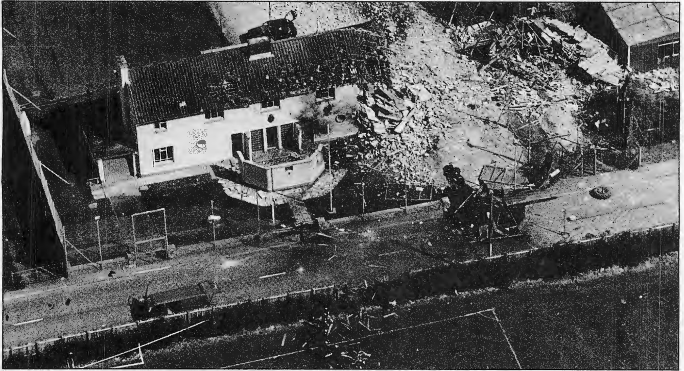
Loughgall Police Station after the attack during which eight IRA men died in an SAS ambush. The damage caused by the massive explosion can be seen as can the closed minibus in which the gunmen tried to make their escape. Photo: Pacemaker Press International, Ltd.
