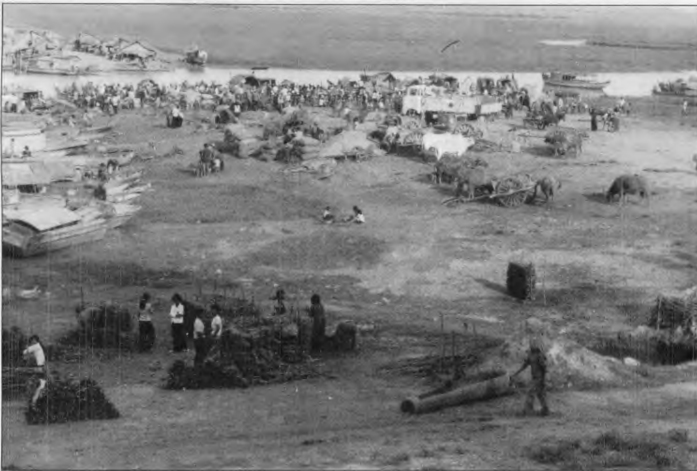
Prey Veng is the site of major construction as the Cambodians struggle to rebuild their country.
