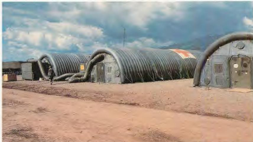
**ABOVE:** Inflatable MASH hospital takes six turbines burning chopper gas to keep it up.
