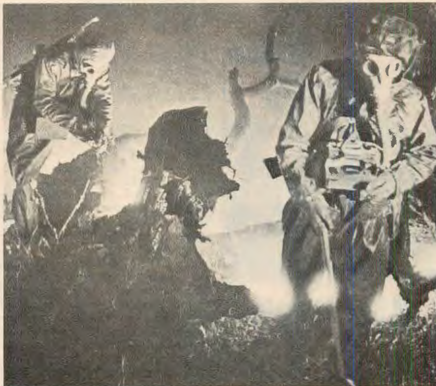
Horror-movie set of Sov chemical training; Military Chemical Forces troops move through glowing wasteland with VPKhR chemical sensors. Chemical troops cannot be expected to work and wear standard OP-1 suit, so they are issued L-1 protective suit in light butyl-covered fabric. Photo courtesy David Isby
