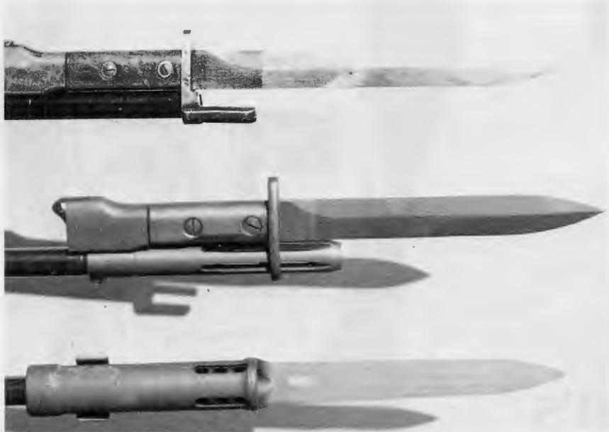
**FAL bayonets: (top to bottom) early bayonet with flash suppressor prongs for plain barrel, same blade and handle but guard modified to accept "American-style" suppressor, and current issue, single-purpose, tubular-handle bayonet for FAL/LAR flash suppressor/grenade launcher.**
