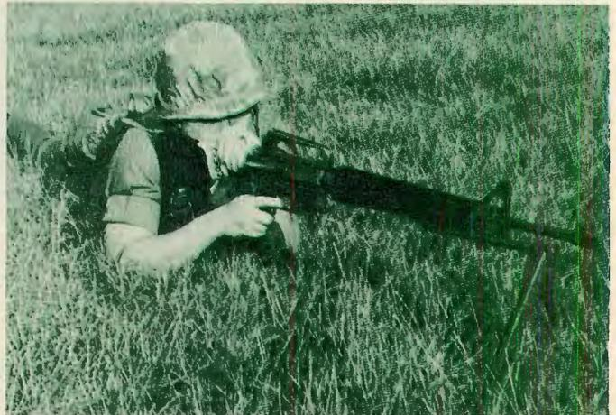
Below: Modified M60 machine gun firing position with bipod standoff device and hinged shoulder rest combination. (Photo credit: Infantry Magazine.)
