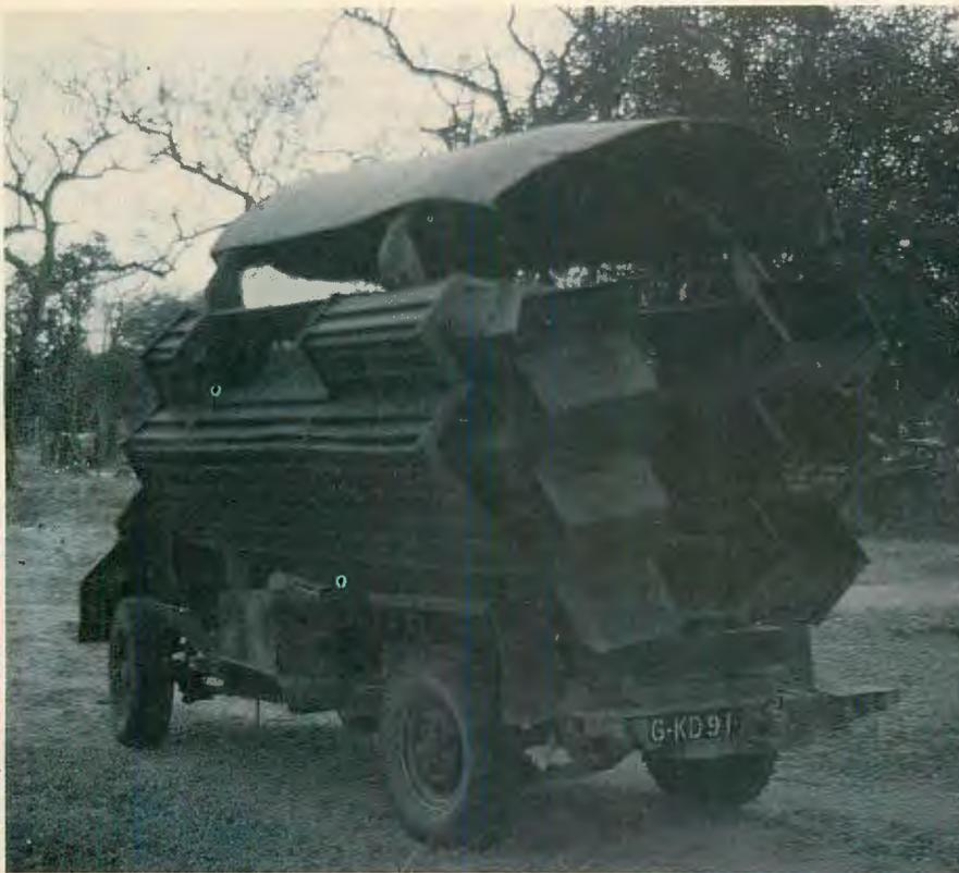
This vehicle has been mine-proofed; armored. Built on a commercial chassis. Used to transport patrols in bush.
