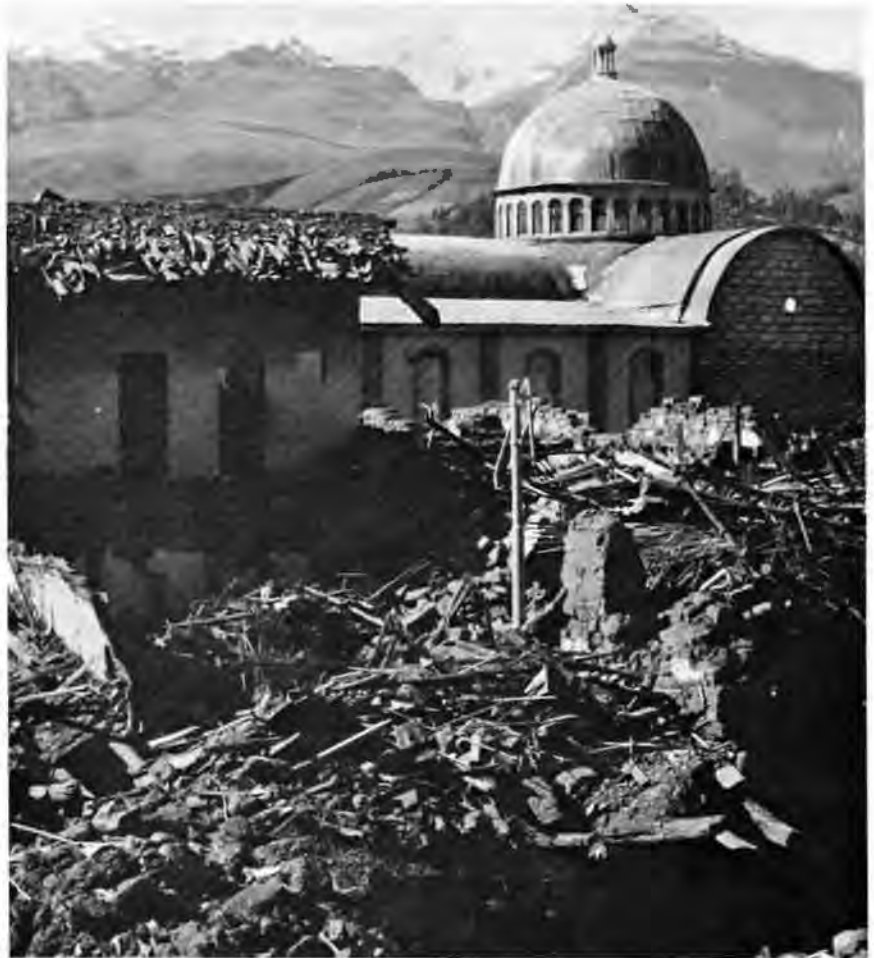
Above: An indication of the damage wrought by the Peruvian earthquake. Over 70,000 were killed in a few hours.
