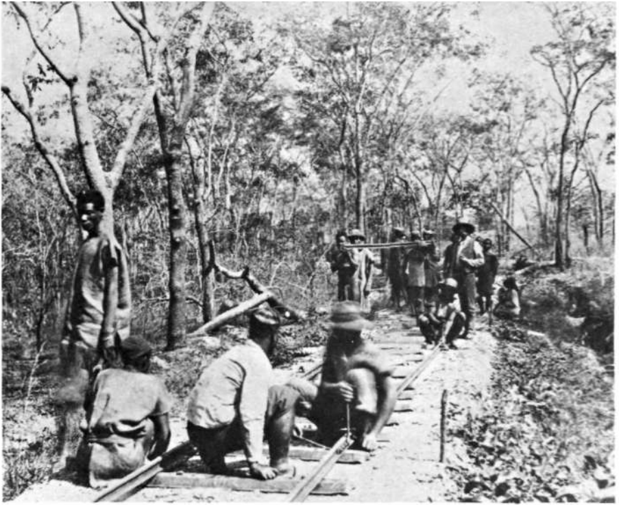
Beira Railway, Plate laying.
