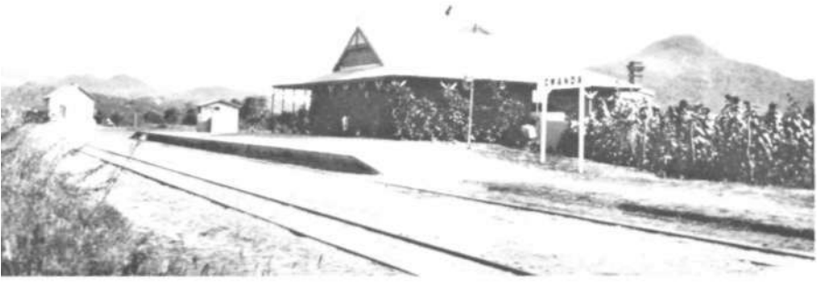
The first Gwanda Station
