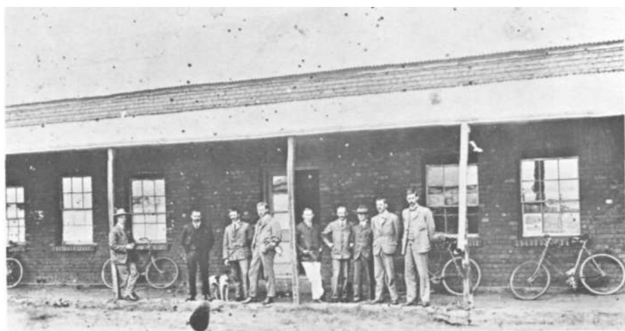
Fig. 3. The staff, in 1907, showing the detail of the windows.
