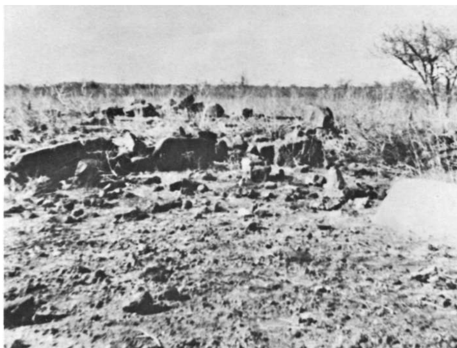
Foundations of the hotel—Tuli. (Photo: National Archives)
