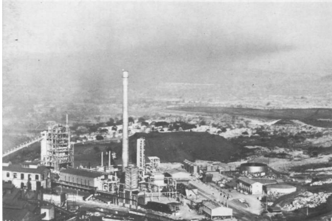
The $8 million coke oven complex which was officially opened in December, 1971, by President Dupont.
