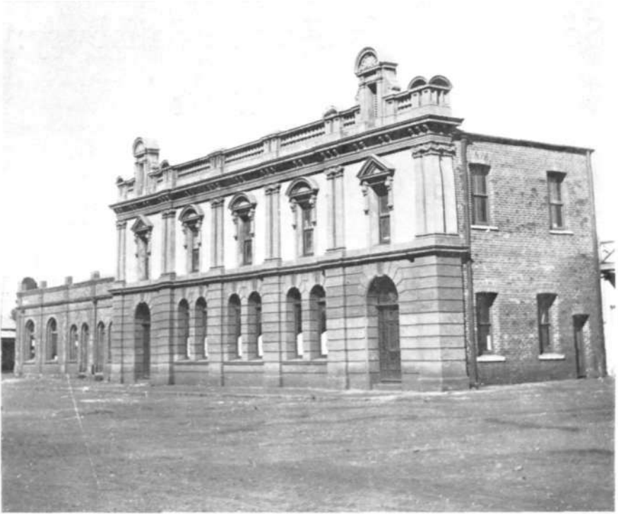
The old Rhodesia Herald building. This building in Victoria Street is a good example of Edwardian artisan workmanship. On the opposite corner stood the first department store, that of Edward's Emporium.
