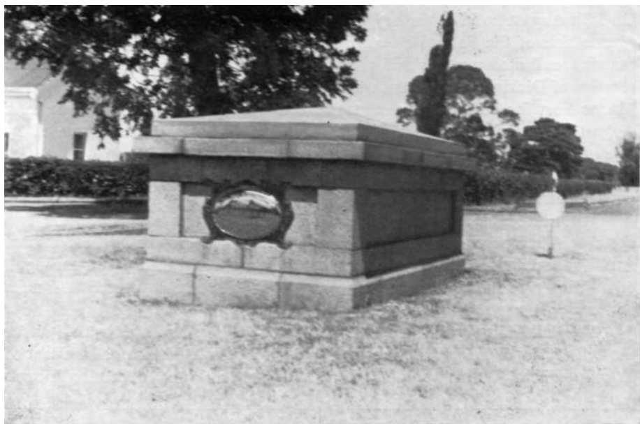
The vault in the Salisbury Cemetery.
