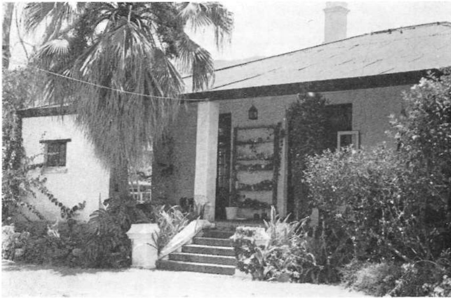
“Three Steps”—Mrs. Fisher’s Residence.
