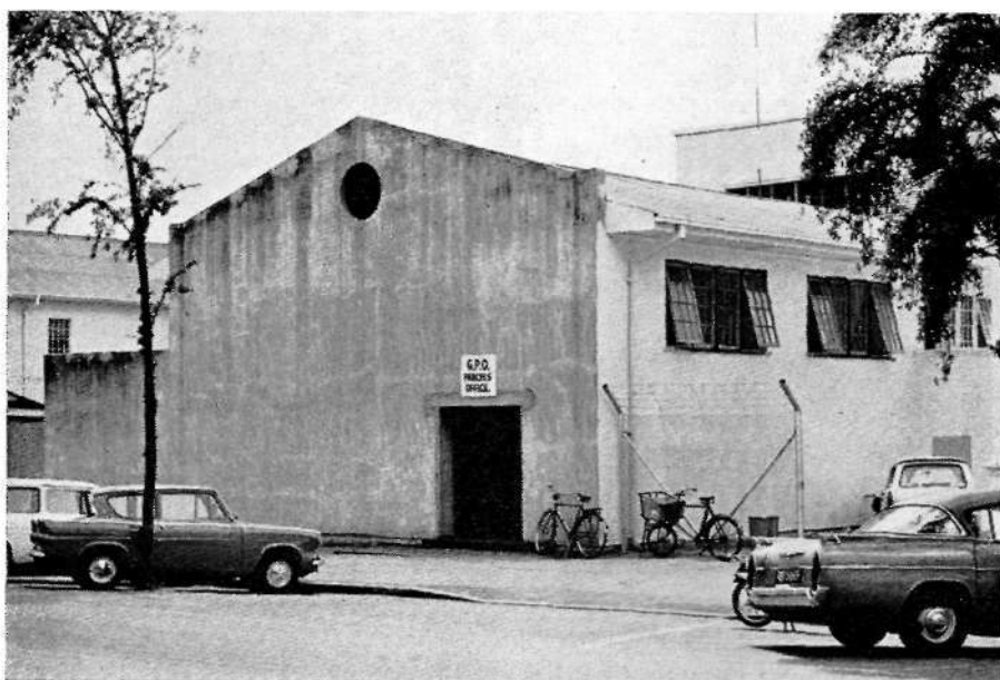
Earliest part of the third museum erected in 1910. The doorway shown was made in 1967, the original entrance having been off the picture on the right.
