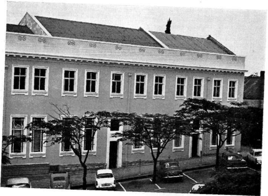
The Chamber of Mines building today. The rusticated stonework and foundation stone assisted identification of detail. (Bruce MacDonald)
