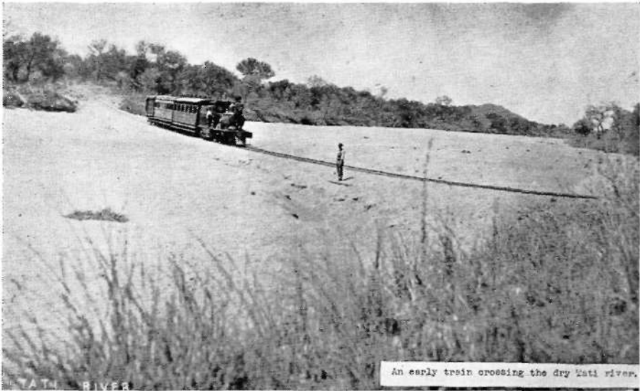
In a concerted effort to reach Bulawayo before the rainy season, 1897, the line north of Mochudi was of a pioneer character—unballasted and unbridged. A passenger train crossing the Tati river bed near Francistown.
